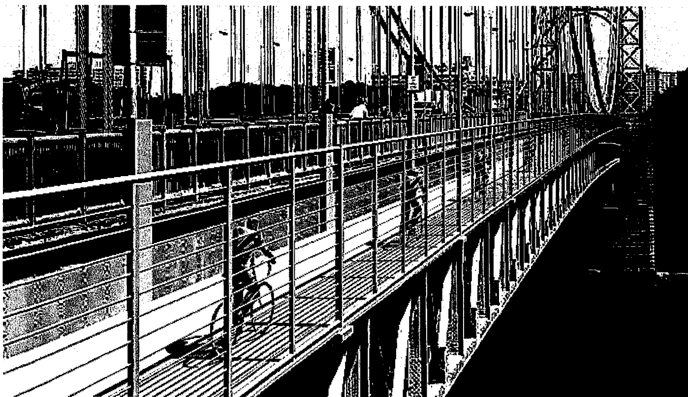
Complete George: (2) 10' paths for cyclists plus (2) 7' paths for peds-runners. 9' anti-suicide barrier.
